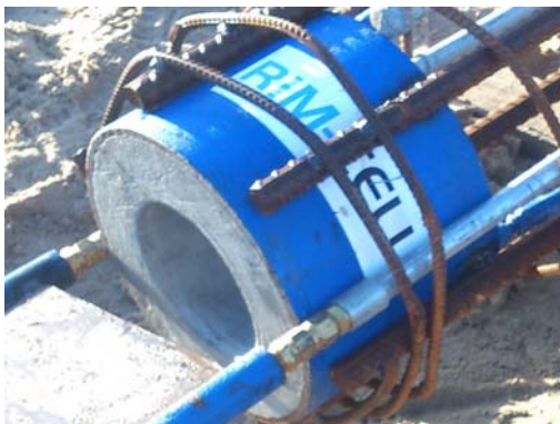
RIM-cell Attached To Reinforcing Cage
