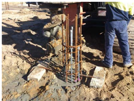
Completed Pile Construction
